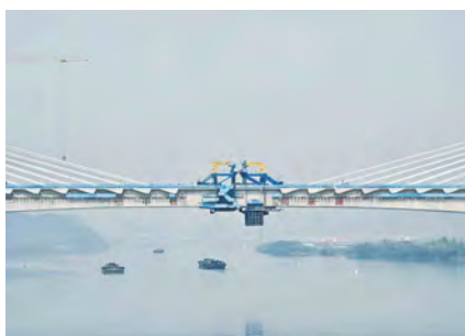
Changtai Yangtze River Bridge 常泰长江大桥
