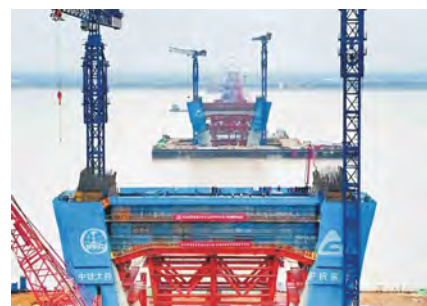
Shanghai Nantong Yangtze River Bridge 沪通长江大桥
